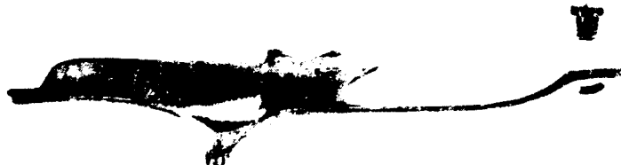
FIGURE 12. INTERRUPTER-EJECTOR FOR RIFLE M1891.
